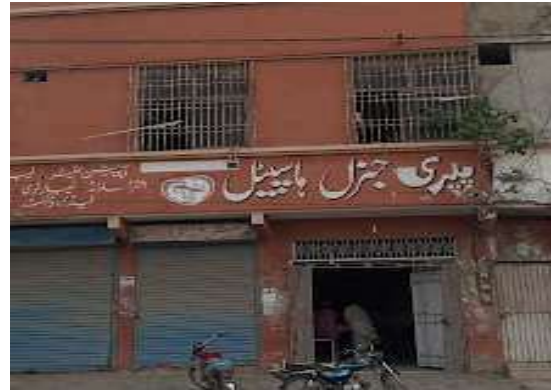
General Hospital in Pipri Settlement
