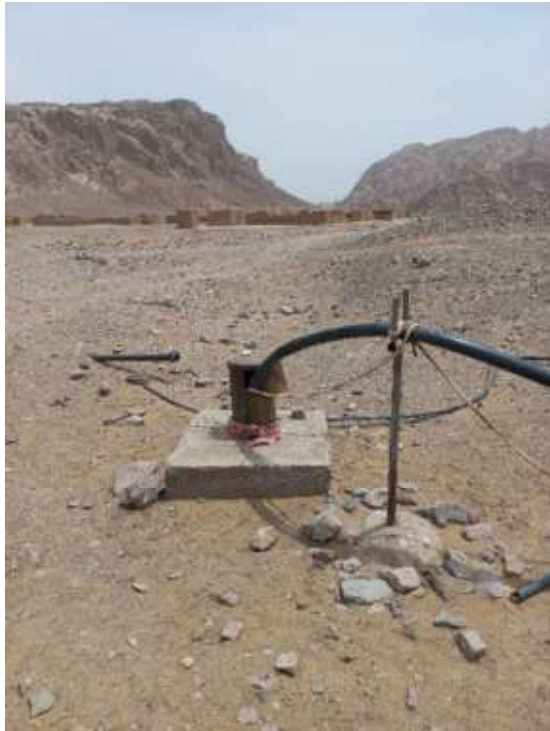
Borehole at W1 – Humai
