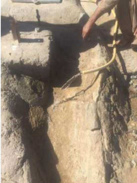
Dug well at W16 – Nok Chah
