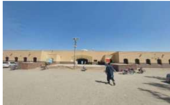
Health Facility in Dalbandin
