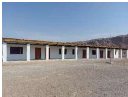
Primary school by RDMC at Humai settlement (East of the Reko Diq Mine Site)
