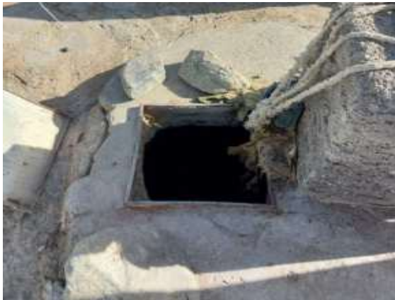
Dug Well for irrigation of palm trees at Humai Settlement
