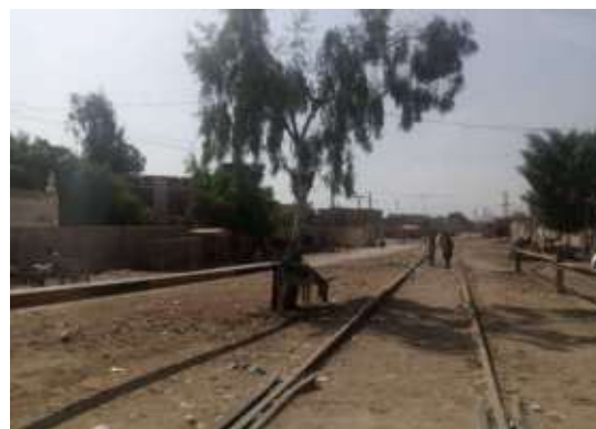
Railway Track near Dadu
