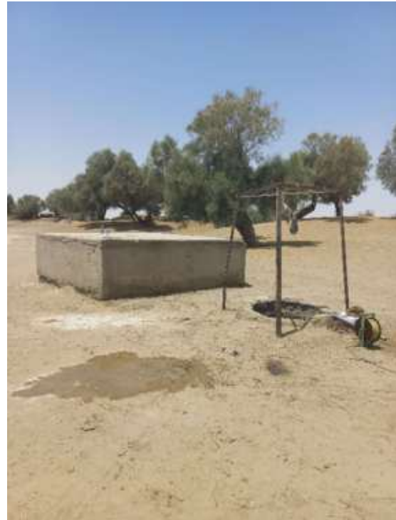
Dug well at TW1– Thul
