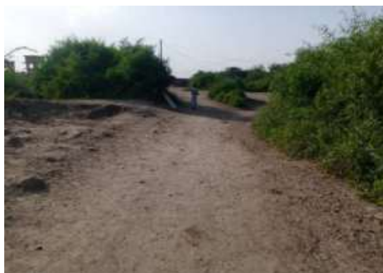
Un-sealed road at Kotri
