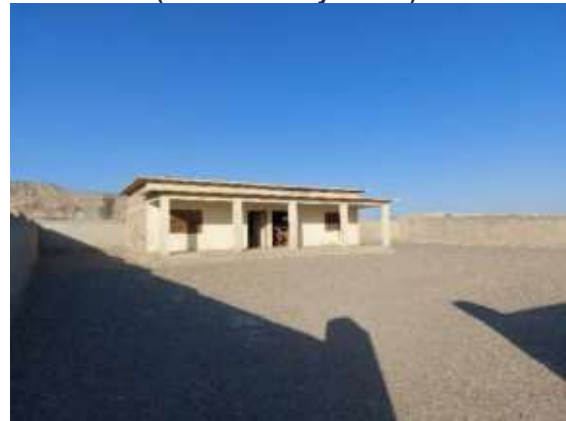
Primary School at Washab Settlement
